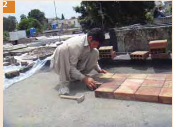
2 Lay Fire clay hollow tiles with out any mortar. Make sure fire clay tiles are laid and set properly.
