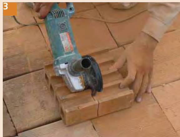
3 Always use tile or marble cutters to cut the tiles where smaller pieces are required. Using chisel for cutting may cause tiles to be broken and wastage of tiles.
