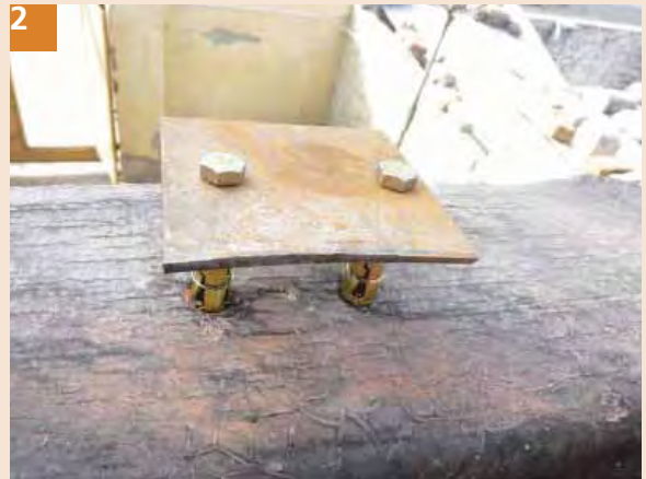
2 Fix MS plate by tightening screws. Do not use hammer to drive the screws.
