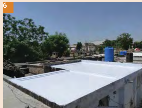
6 Avoid walking on freshly painted surface. Cover the surface in case of any possibility of rain splashes or storm winds.
