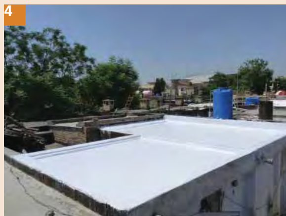
4 Let the surface dry for minimum two hours after the application of first coat. Do not allow anyone to walk on freshly painted surface.
