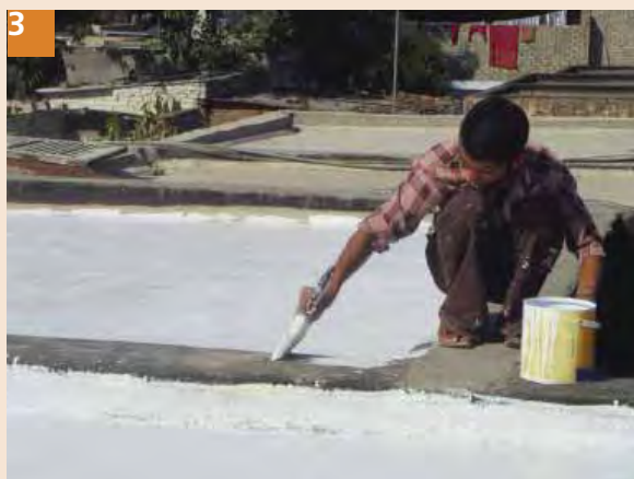
3 Corners and edges are painted in the end to provide ease in work. Use brush for painting in corners and edges.
