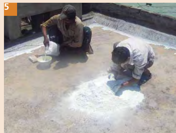
5 Mix OCEVA-MOL chemical with white cement in required proportion i.e. one part of chemical and two parts of white cement.
