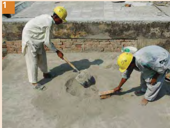
1 Clean the surface and prepare cement sand mortar (1:4). Sand should be free from mud, water should be clean and free from impurities.
