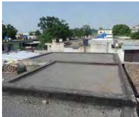
View of roof top with 370 sft
