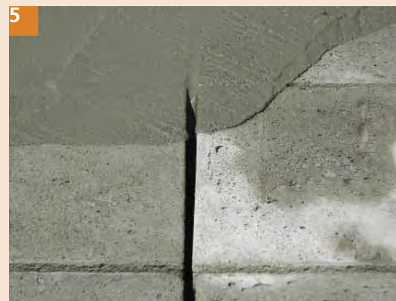
5 Use cement slurry for grouting. Use trowel to properly seal the gaps between tiles so that water may not penetrate from the joints.
