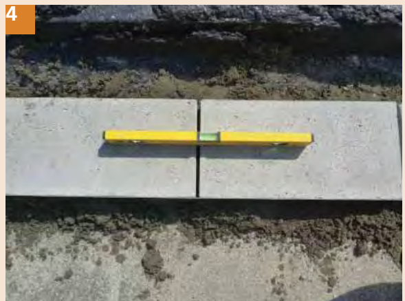
4 Lay tiles in level with a gap of 1/2 inch in between for grouting. Remove surplus mortar around the tiles.
