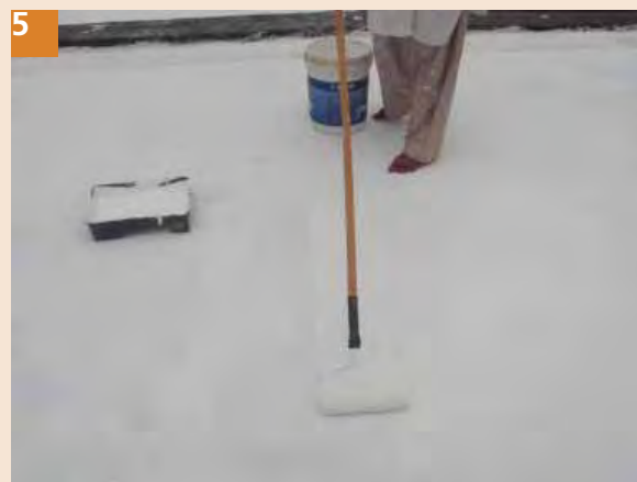
5 Apply second coat by moving backward from the front. Shoes or bare feet should be clean and it should not left a mark on the surface.
