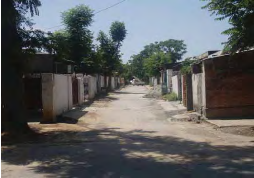
Houses on the left lane of the street have a roof project area of 570 sft each.
