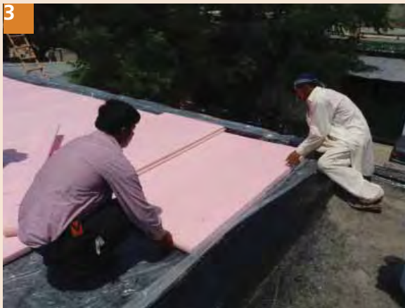
3 Lay the 2 Inch thick foam (extruded polystyrene sheets) on the plastic sheet. Do not damage the foam. Provide 1 inch overlaps where there are joints to avoid gaps.
