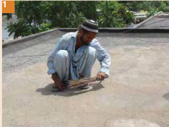
1 Clean the roof surface. Remove dust, pebbles, scratch bitumen or concrete humps if any to make the surface even and smooth.
