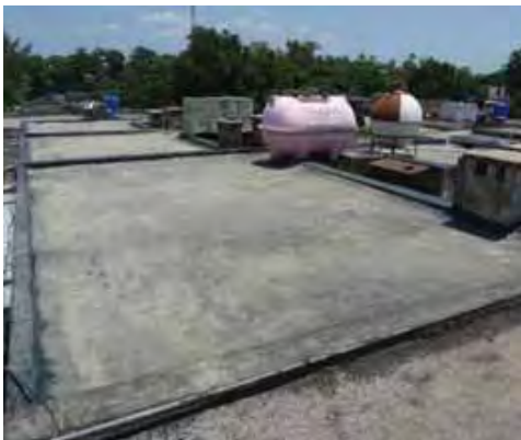
View of roof top with 570 sft
