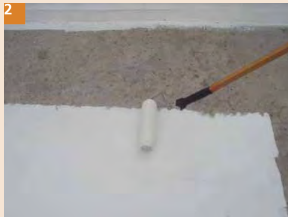
2 Apply first coat of enamel paint with the help of paint roller if the roof area is larger, brush can be used for smaller roofs.
