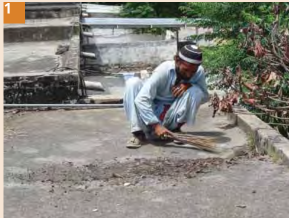
1 Clean the roof and remove dust, pebbles, leaves etc from the surface.
