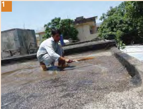
1 Remove the loose particles, pebbles and dust from the roof surface
